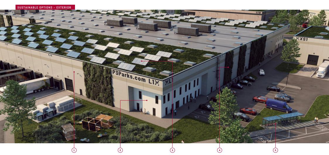
We will continue to upgrade standing assets with energy efficiency measures, such as LED, right-sized HVAC, increased insulation, and energy storage technology and building out our developments to the best possible specification.
